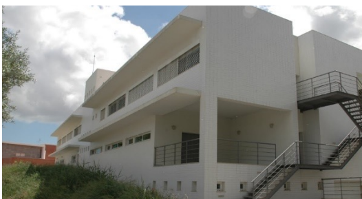
Figure 32 - School Building of the Pulido Valente Hospital
